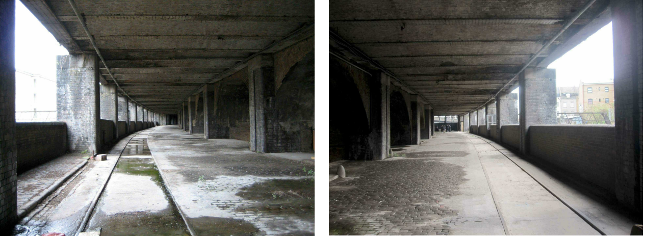
JACK ARCHED LID TO LONDON ROAD - This significantly contributes to the character of London Road and is generally to be retained and repaired.
